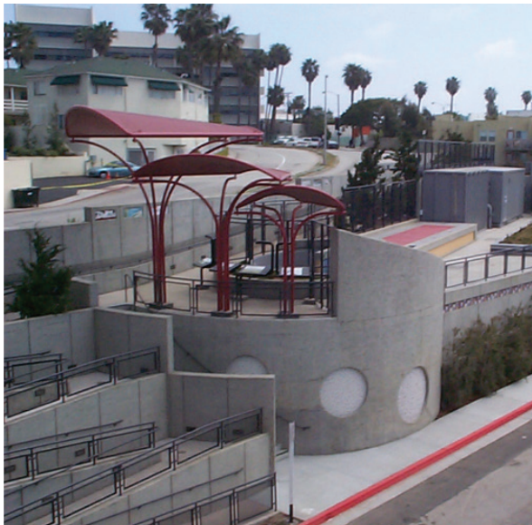
The Santa Monica Urban Runoff Recycling Facility collects, treats, and reuses approximately 500,000 gallons per day of urban runoff.
