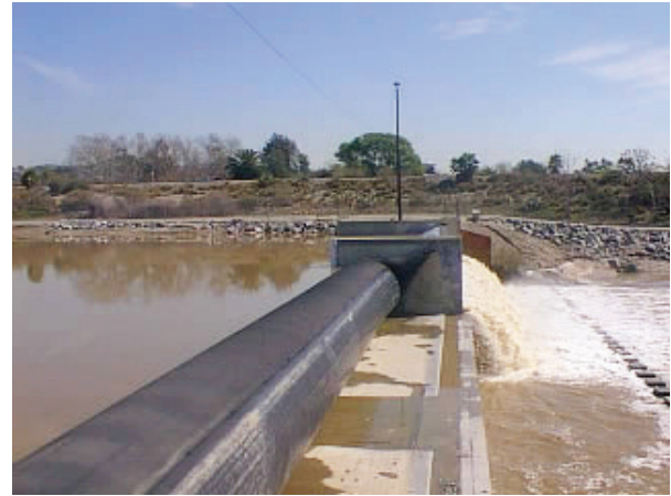
LACFD operates inflatable dams on the San Gabriel River to promote short-term in stream recharge.
